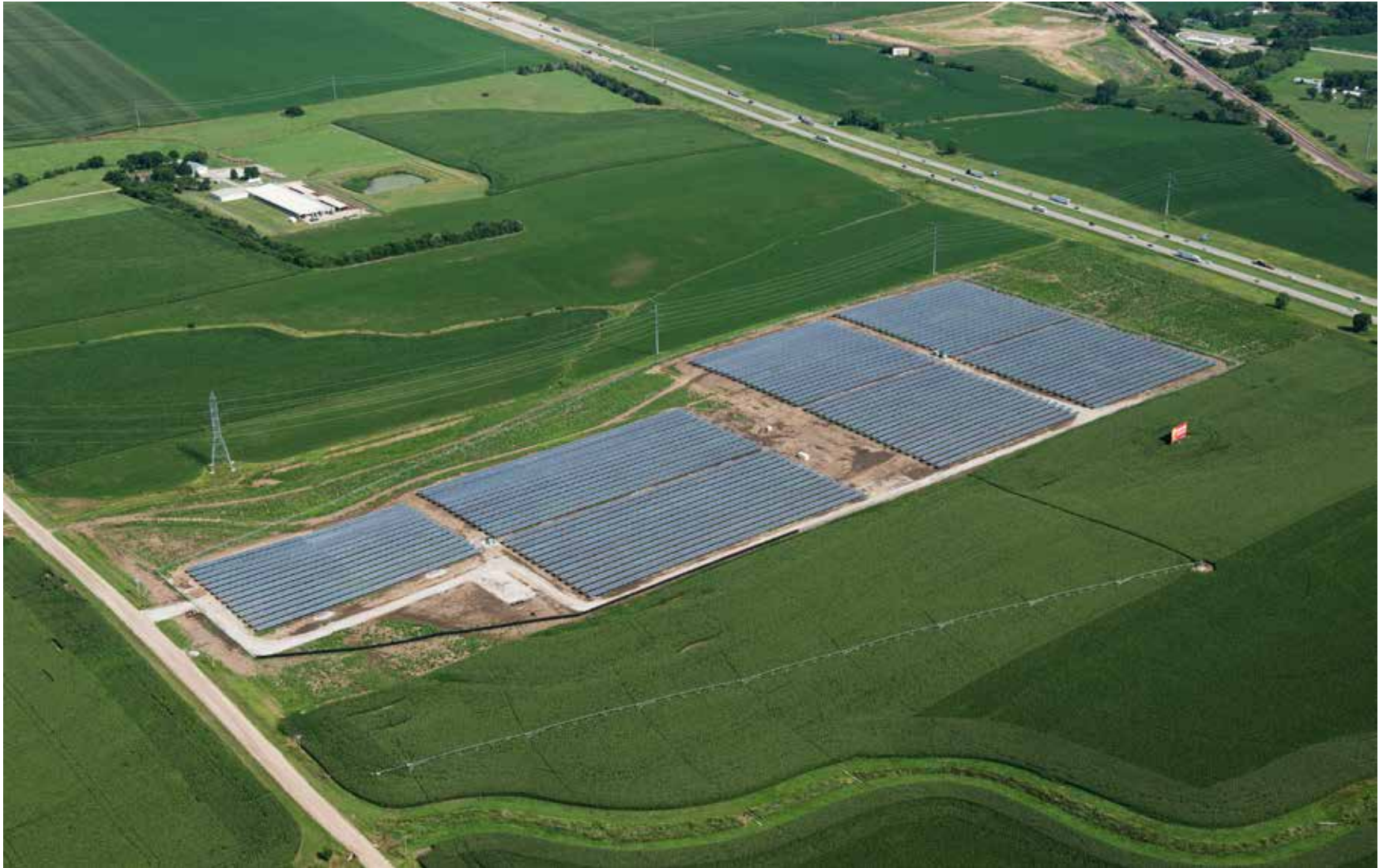
Aerial view of the completed project.
