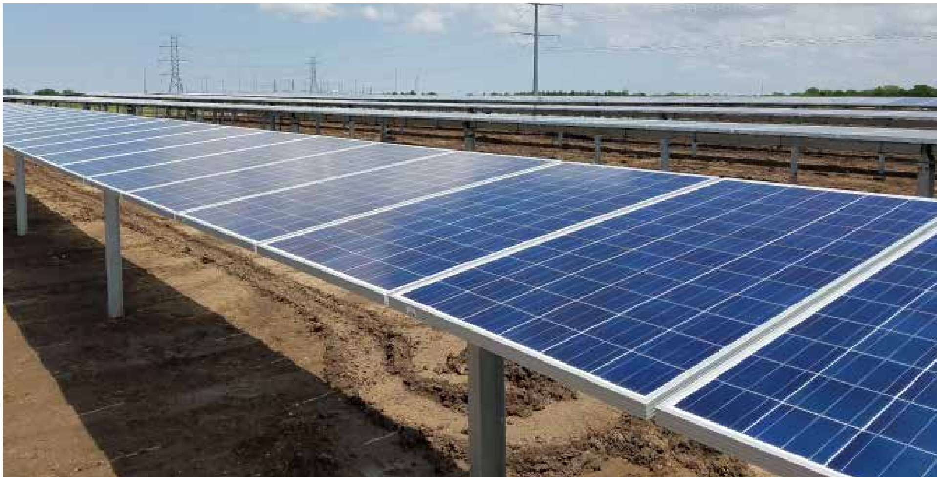
Installation progress of solar panels and tracking assemblies across the site.
