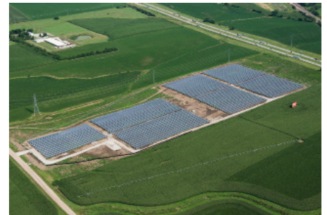
LES' community solar project, located at Northwest 75th & West Holdrege streets, generates 5 MW DC of solar energy.
