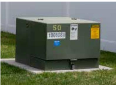
*LES pad-mounted transformer with proper clearance.*
